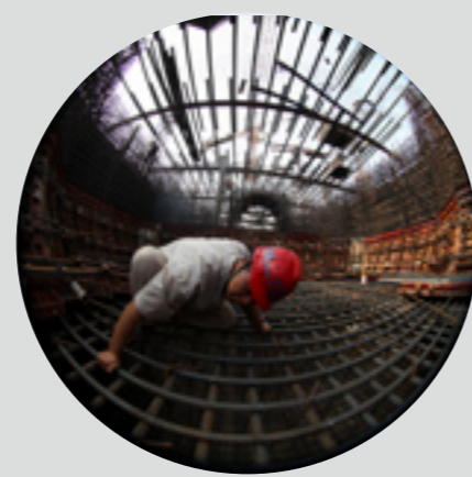
7#墩0#块钢筋自检
